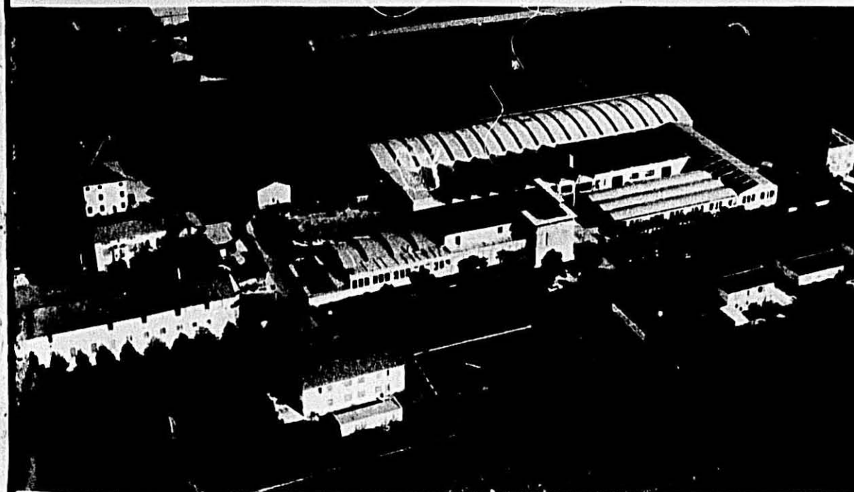
Air view of Pavan works
